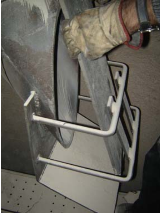
Figure 6 – Cyclone Dipleg Check Valve
